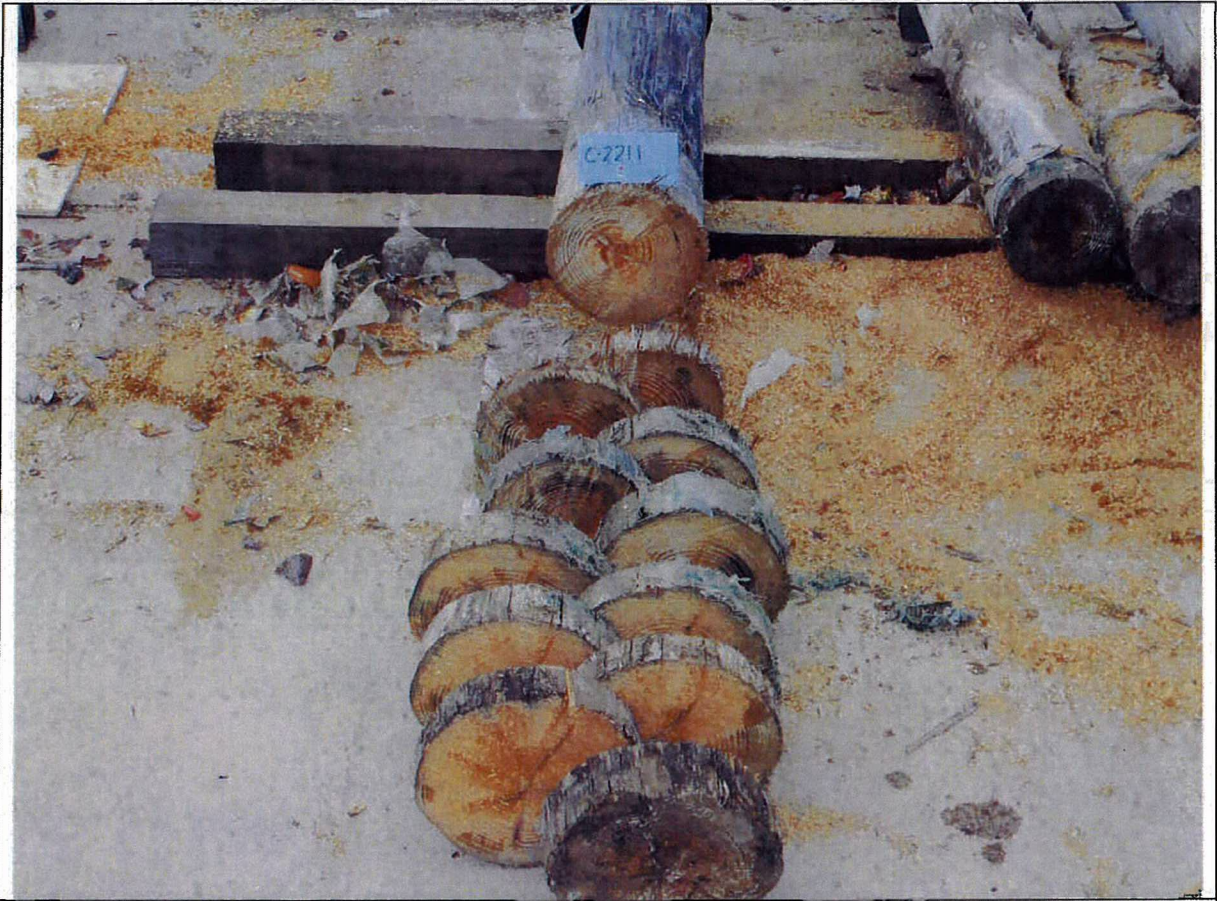
Figure 10 – Pole #2211 had internal decay surrounding the pith from the bottom up to approximately 24”.
