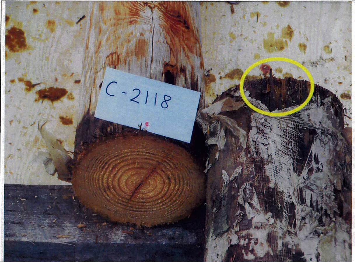
Figure 9 – Pole #2118 did not show any signs of internal decay underneath the small spot of surface decay.
