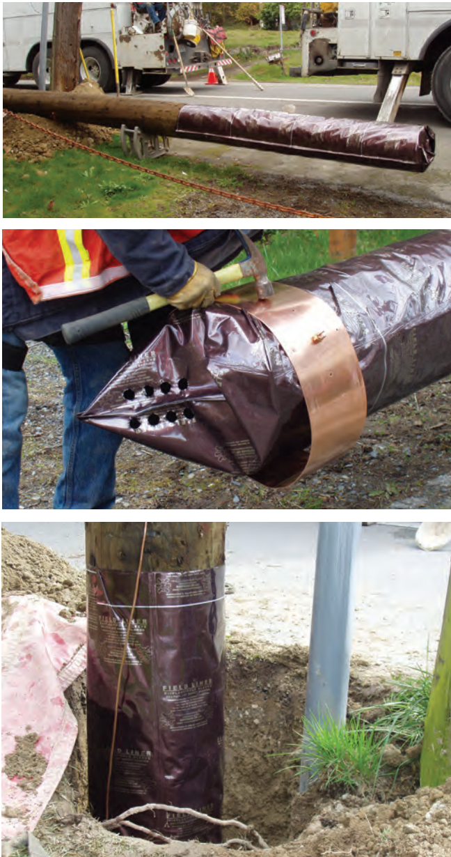
Figure 12. Example of a commercially applied pole barrier used to protect the belowground portion of a pole.
