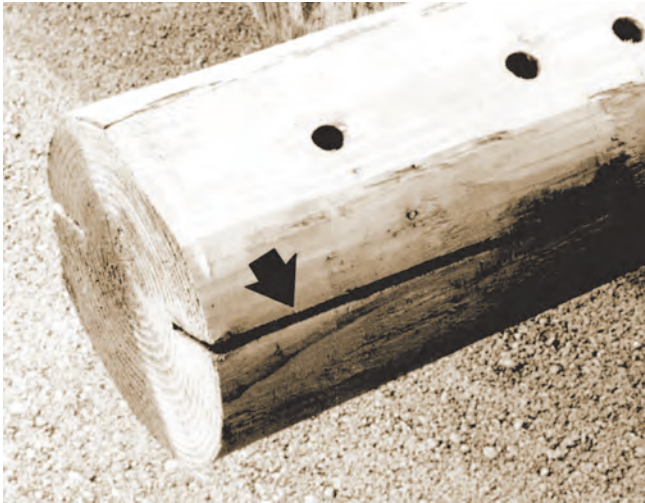
Figure 7. Kerfing (arrow) can be used to control checking of poles, thereby reducing internal decay in service.
