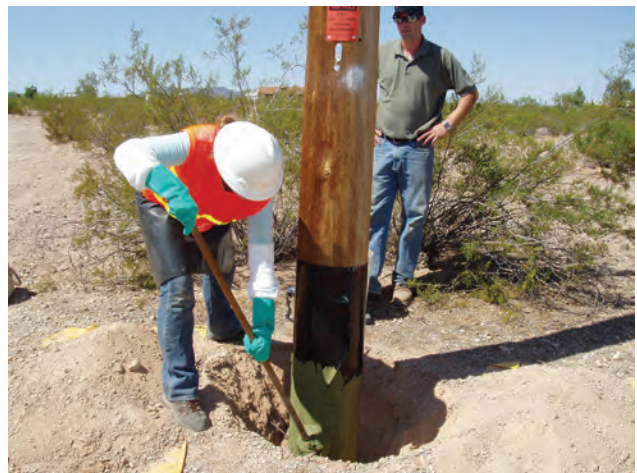
Figure 45. Applying groundline treatment.
