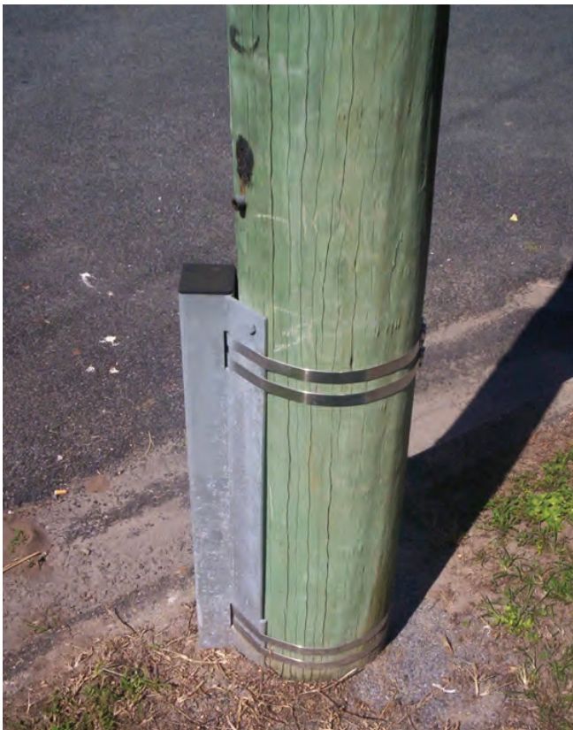
Figure 33. Examples of steel trusses used to reinforce deteriorated poles.
