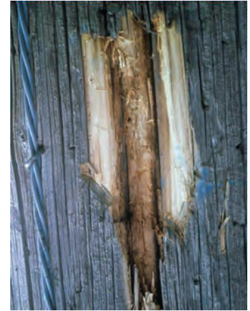
Figure 14. Weathering of a cedar pole turns the surface grey, but the wood underneath is unaffected.
